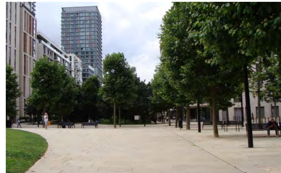
Victory Parade looking West towards Portlands showing a expanse of hard landscaping.
